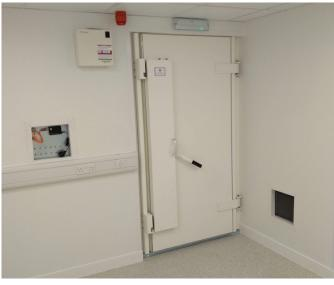
The NTD-S100 system is a very versatile shielding system which offers a vast range options for configuration and modification and is in fact full demountable and able to be relocated and changed in size and configuration to meet your future requirements.
